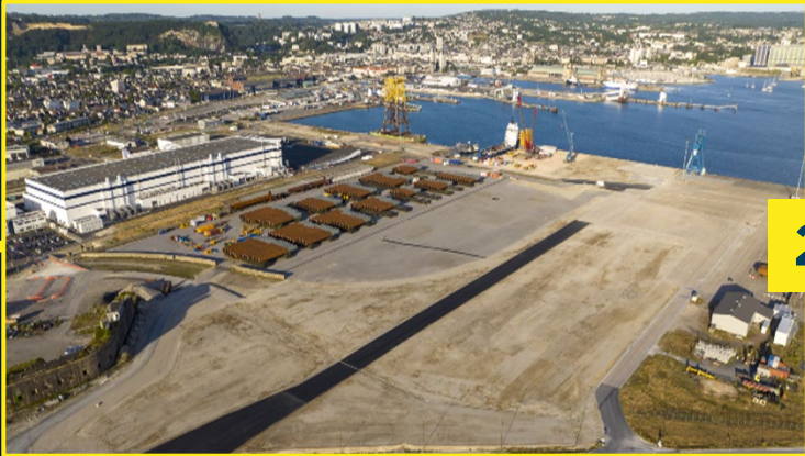
Cherbourg: fitting out an installation hub
