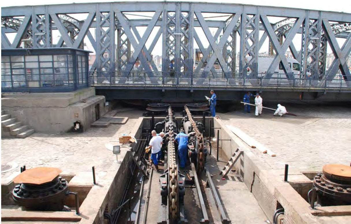
Port of Dieppe – Pont Colbert ©Ports de Normandie
